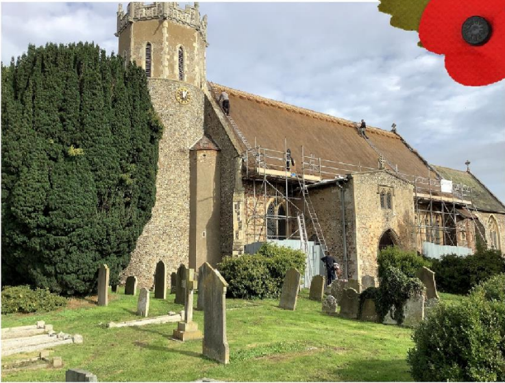
Thatchers completing the Acle Thatch repairs.
